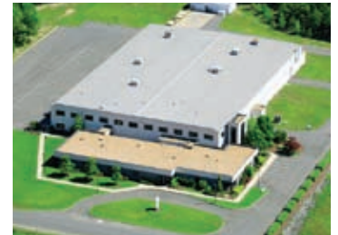
Walter's 65,000 sq ft facility in Virginia. We also have offices in Dayton, OH, Los Angeles, and Mexico City
